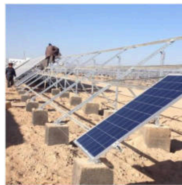
GROUND-MOUNT STRUCTURE AND MODULE INSTALLATION
