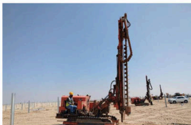
PILE DRIVING AND SETTING OUT FOR A GROUND-MOUNT ARRAY, STAGE 01
